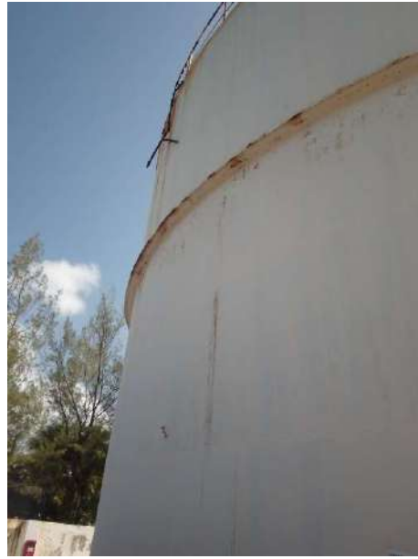
Areas of Rust on External Tank Shell
