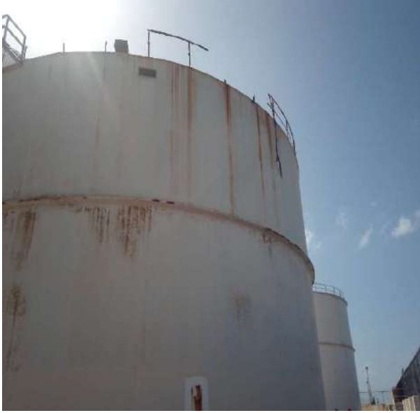
Areas of Rust on External Tank Shell
