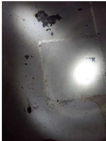
Tank #32198 Bottom Plate Failure
