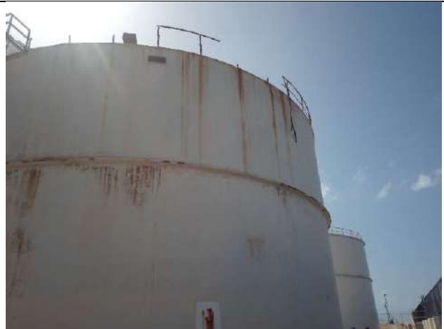
Areas of Rust on External Tank Shell
