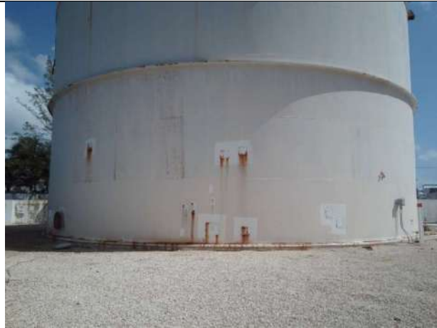
Areas of Rust on External Tank Shell
