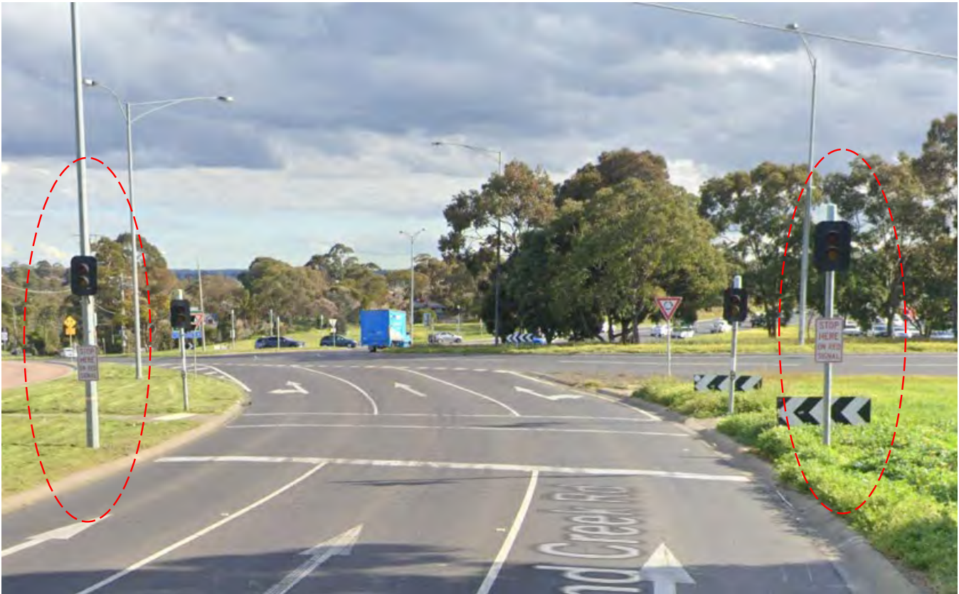
Traffic metering signal in dark mode during off-peak periods
