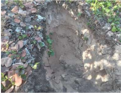
Photo 1 – Trial Pit No. 1 Dug.
