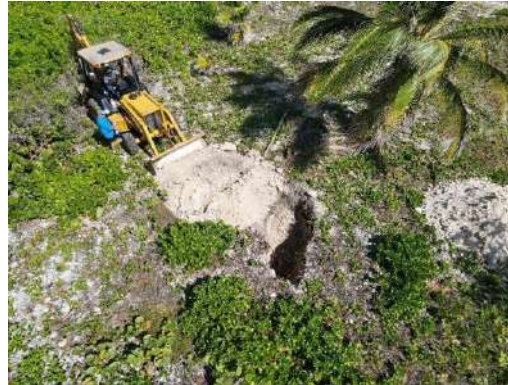
Photo 12 – Backhoe Refilling Trial Pits.
