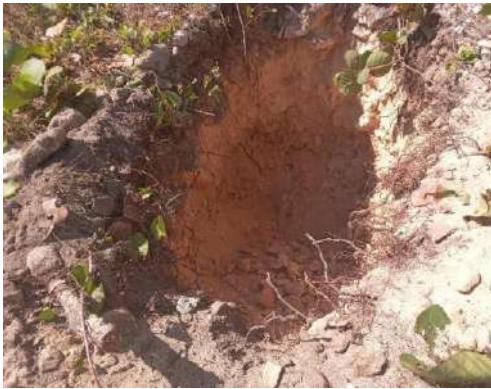
Photo 7 – Trial Pit No. 4 Dug.
