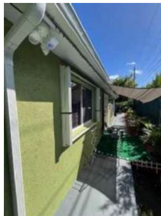
Back of ATF unit
