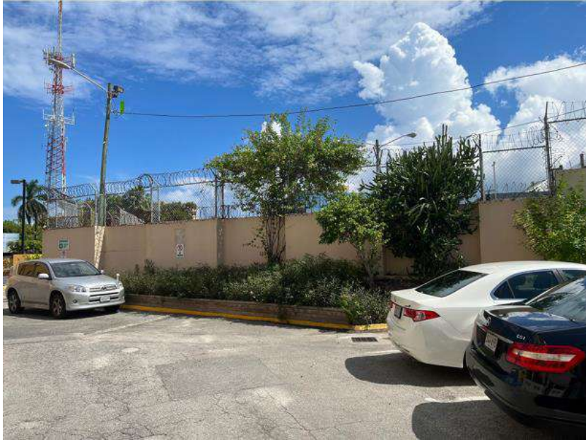
Figure 1: Barbed wire and razor wire above the wall and chain link fence at the George Town Police Station.
