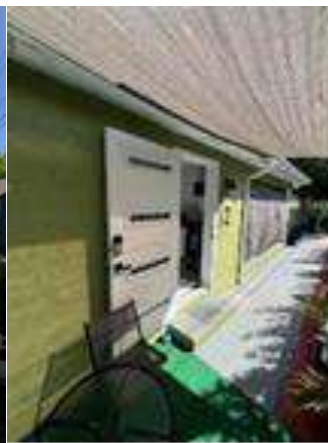
Entrance to ATF unit
