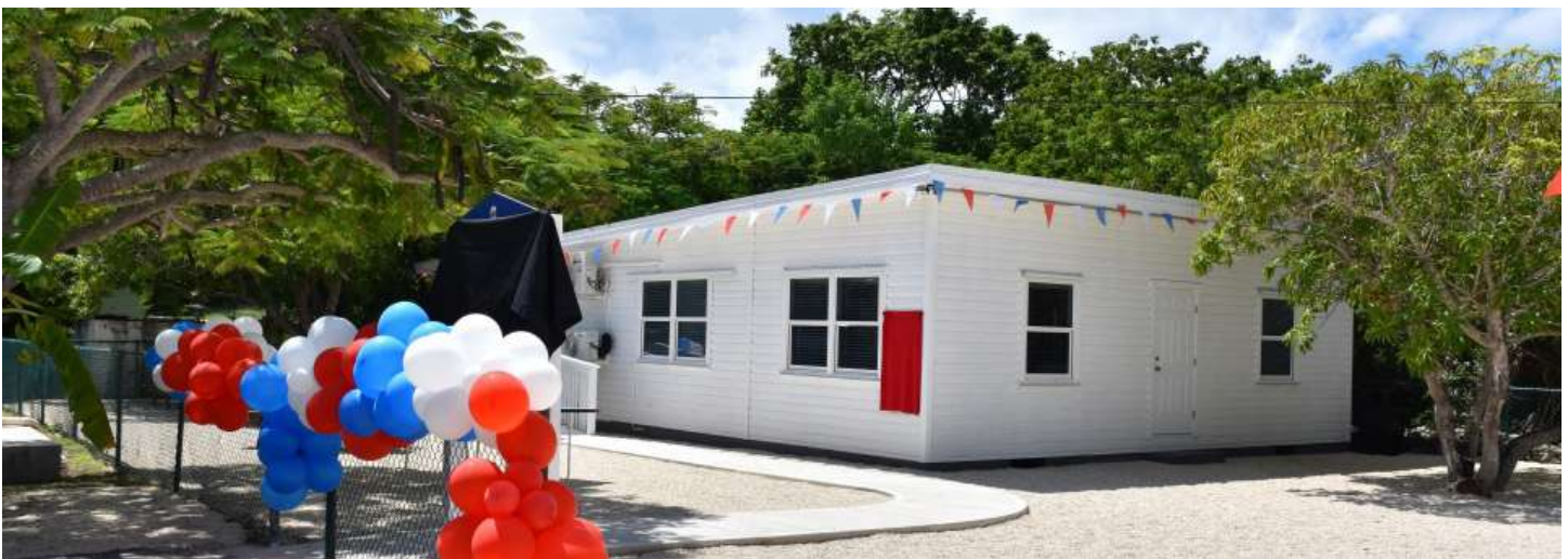
Front exterior view of the Civil Service Learning and Recreational Facility in Cayman Brac)
