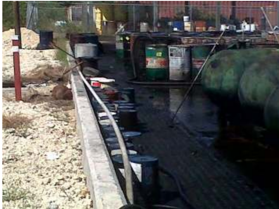
Figure 10 Bunded Waste Oil Storage Area at the GTLF (After Figure 3.2 in Amec Foster Wheeler, 2016c)
