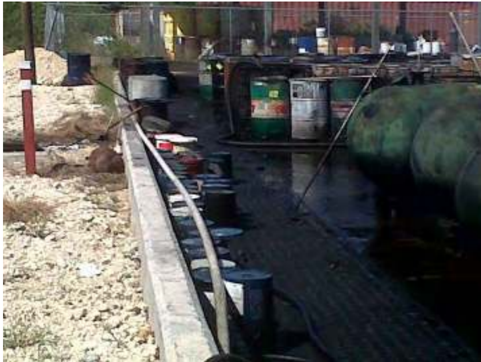
Figure 9.10 Bunded Waste Oil Storage Area at the GTLF (After Figure 3.2 in Amec Foster Wheeler 92 )
