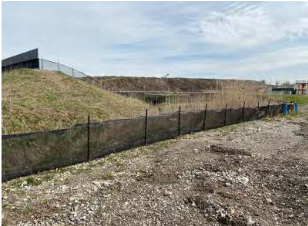
Figure 8 Example of wildlife exclusion fence (fencing on the right side of the figure)
