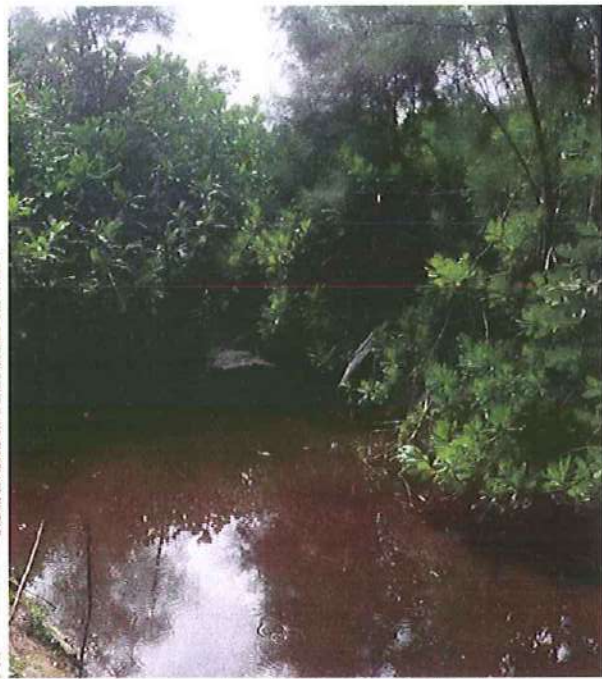
Fig 4: Landward End of South Sound Culvert
