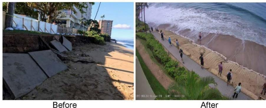
Proposed mattresses deployed along Kaanapali Beach, HI.
