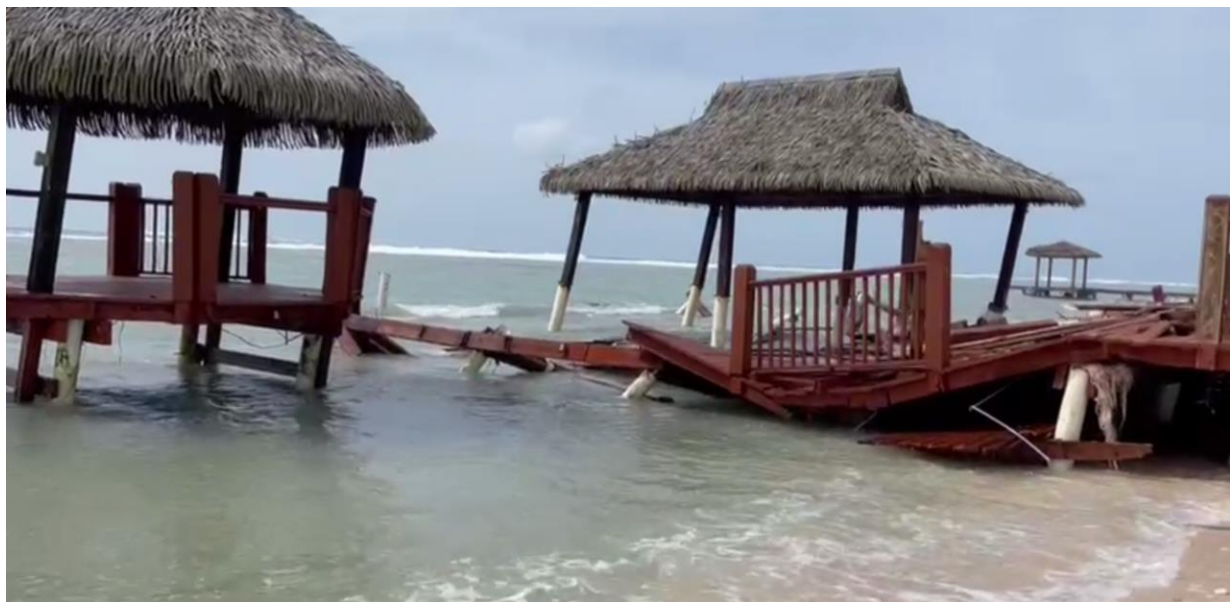
Figure 12. The dock at the White House in Bodden Town is one of the most substantial existing docks in Cayman which was used as a restaurant, and it was damaged during Tropical Storm Grace and debris was scattered along the beach.
