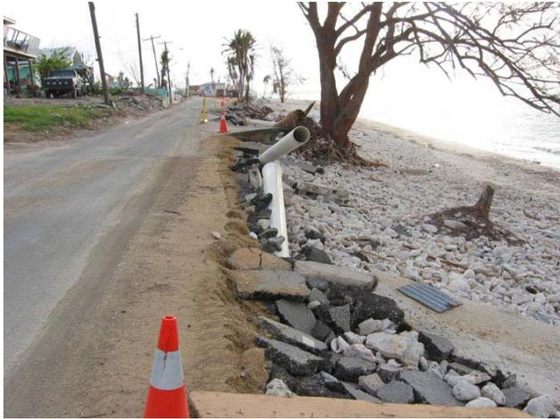
**Photo 10 Water lines along coastal road exposed and damaged. Credit: ECLAC 2005**
