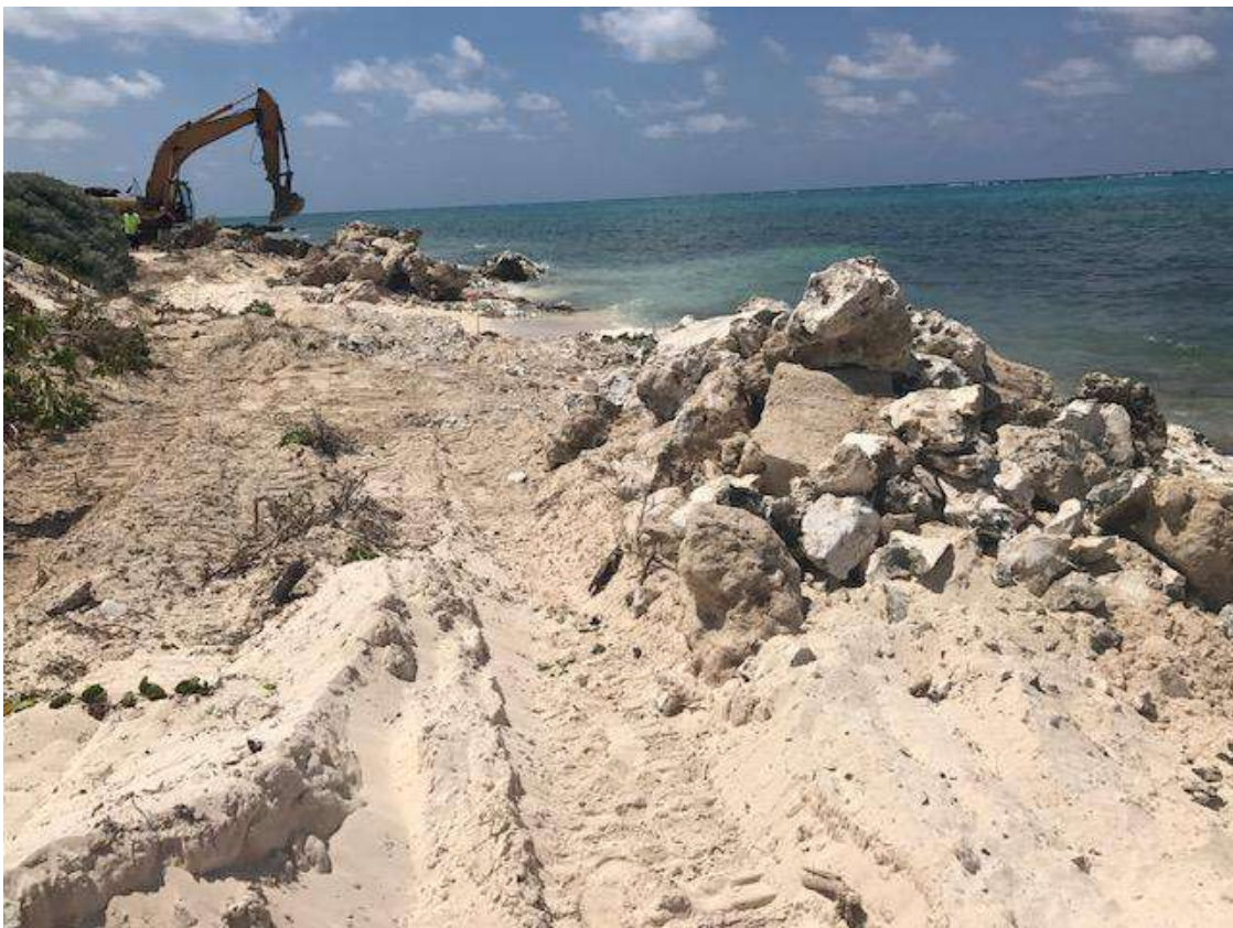
Figure 8. Stockpiling and on-land activities impacting the marine environment through turbidity and deposition of waste
