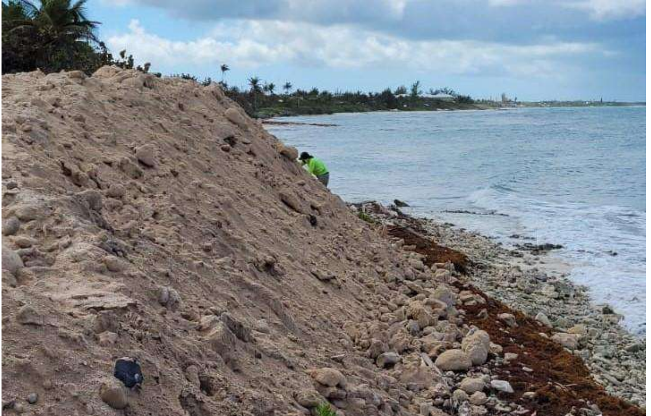
Figure 12. Material stockpiled too close to the water's edge which would or would be likely to enter the marine environment during a storm.
