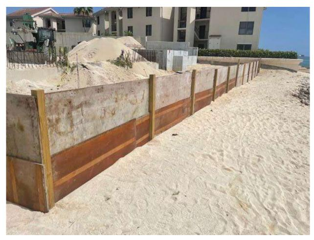
Figure 7: An example of suitable construction fencing to protect turtles (Source: DoE, 2022).
