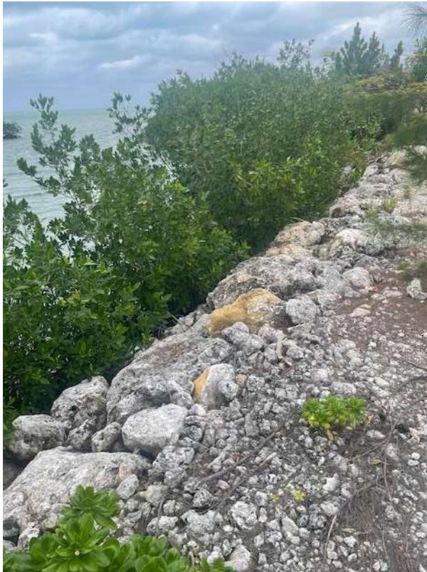
Shoreline: Riprap and Mangroves (Left), Riprap Only (Right).
