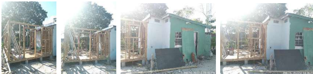
PHOTOS COURTESY OF CE22-0018
