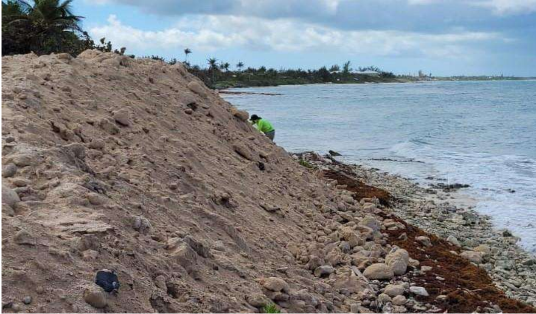
Figure 11. Material stockpiled too close to the water's edge which would or would be likely to enter the marine environment during a storm.
