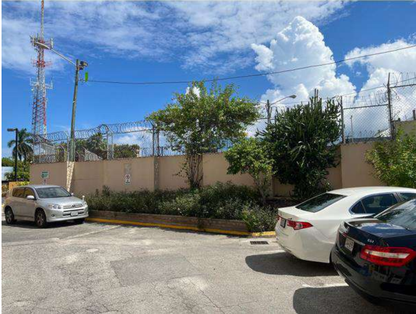
Figure 1: Barbed wire and razor wire above the wall and chain link fence at the George Town Police Station.
