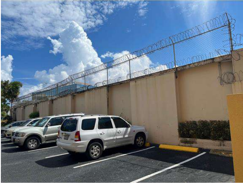
Figure 2: Barbed wire and razor wire above the wall and chain link fence at the George Town Police Station.
