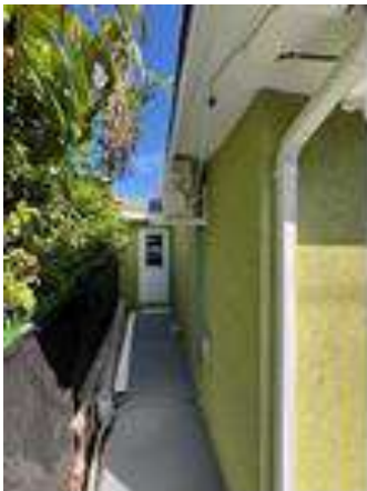
View towards Storage
