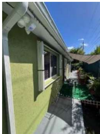
Back of ATF unit
