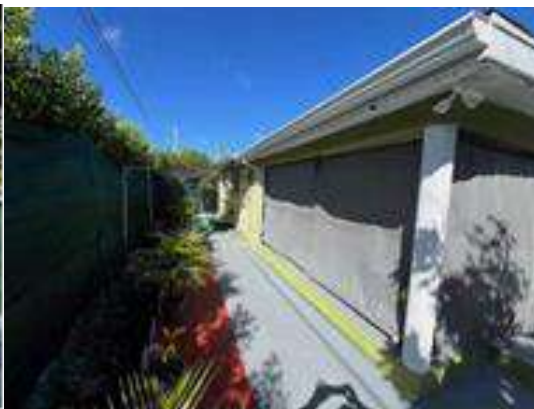
View from South Side towards unit
