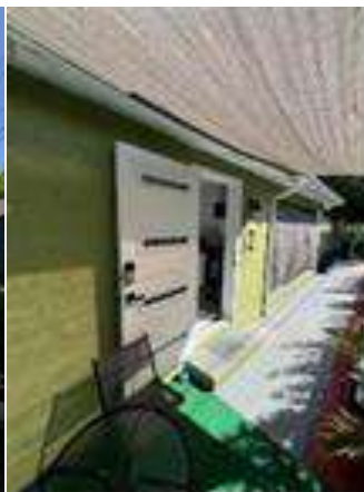
Entrance to ATF unit
