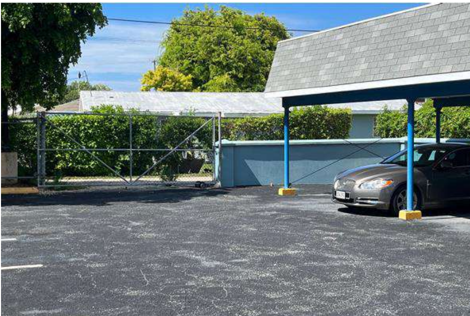
Figure 5: The end of the existing concrete wall at Elizabethan Square.
