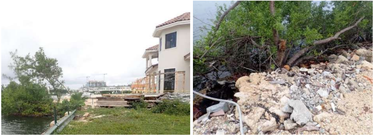
Figures 6 and 7. Loose materials and construction debris being stored on the water's edge, and that material entering into the marine environment.
