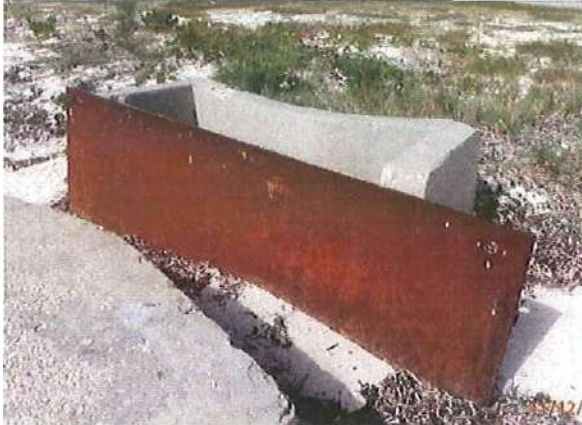
Fig 3: Closed Culvert in South Sound Culvert
