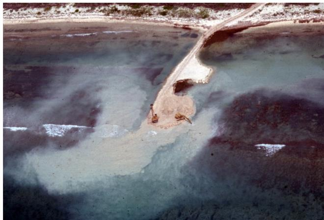
**FIGURE 2: CHANNEL CLEARING BY MECHANICAL EXCAVATORS AND FILL PAD, NORTH COAST, GRAND CAYMAN. (DOE)**
